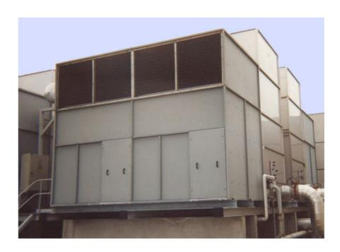
Flow rates : from 70 to 570 m3/ h Cooling capacity : from 1100 to 3 300 kW  $\,$
